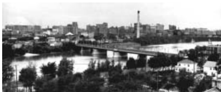
The old Provencher Bridge, August 1952
