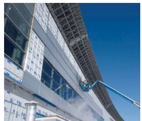
Progress on the Winnipeg James Armstrong Richardson International Airport redevelopment
