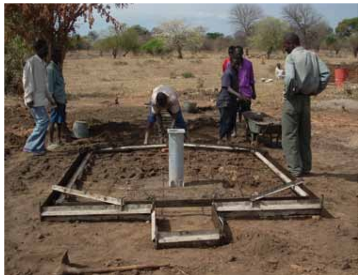
Construction of a well in Malawi
