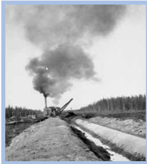
Burying of railway line and aqueduct by steam shovel. Source: Manitoba branch of the American Public Works Association
