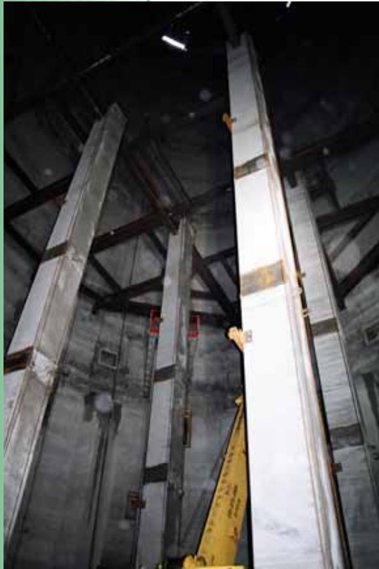
Columns, Terminal, Detroit
