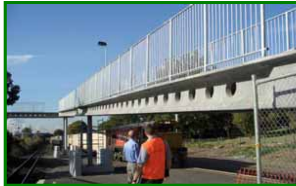
Papatatoe LRT Bridge, NZ
