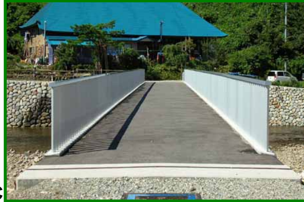
Yamagata Footbridge, Japan
