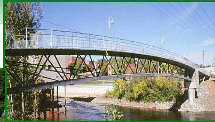
Sherbrooke Footbridge, Quebec
